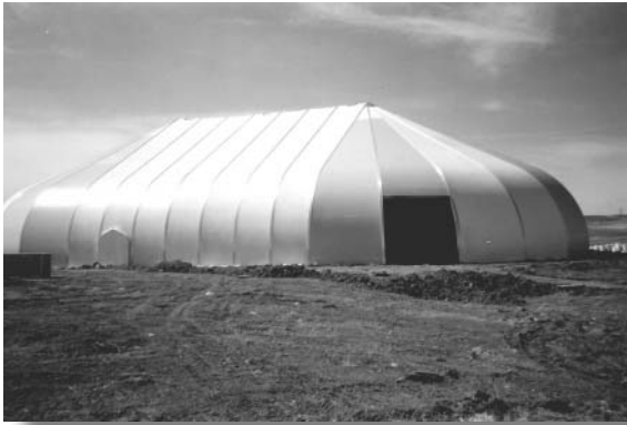
Structure over North Waste Pit to Enclose Attempted Pit Excavation, 1999
