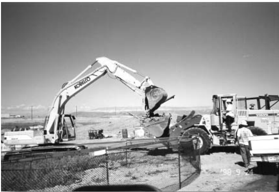
Excavation of Middle Waste Pit, 1998
